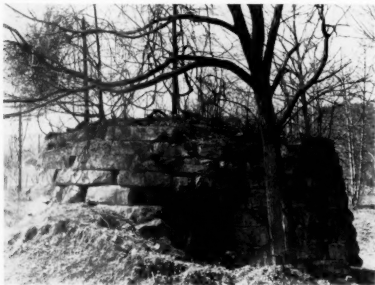
Valley Furnace: Base only remains intact.
